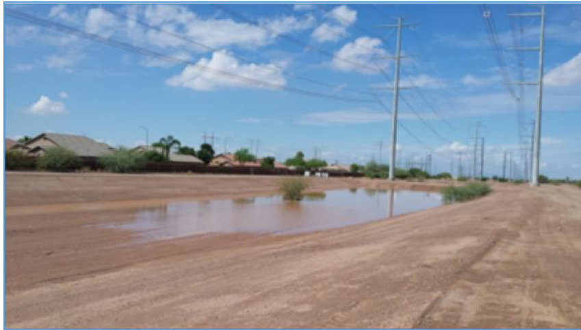
Figure 2: Retention Basins in Transmission Line Right-of-way. Salt River Project. Phoenix, Arizona.
