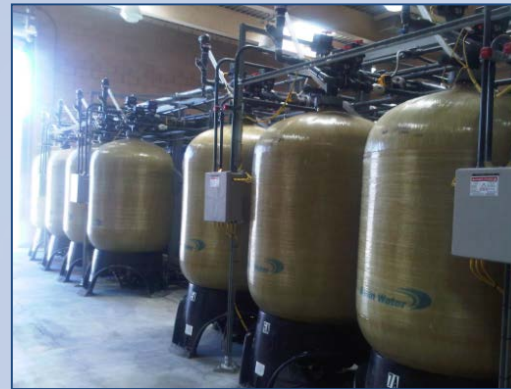
Strong-Base Anion Exchange with Residuals Treatment (SBA)
