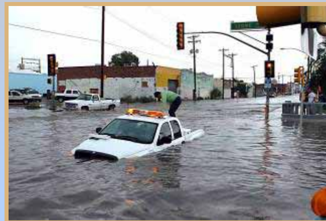
Inadequate stormwater facilities in urban core
