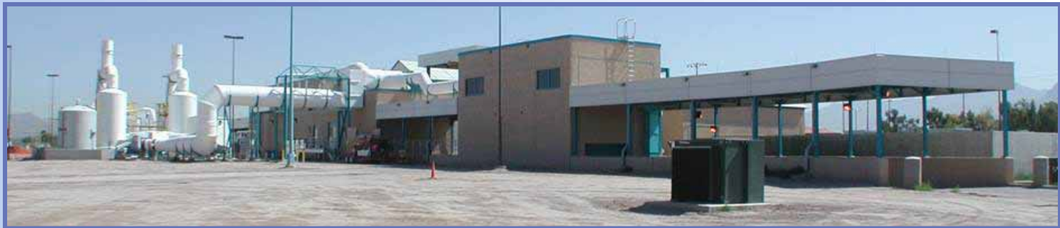
Ina Road Wastewater Reclamation Facility (WRF) Headworks
