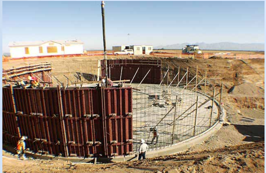
Construction of the Corona de Tucson WRF – Pima County, Arizona
