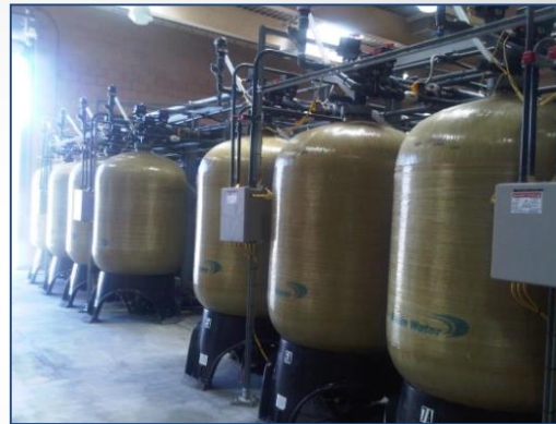
Strong-Base Anion Exchange with Residuals Treatment (SBA)
