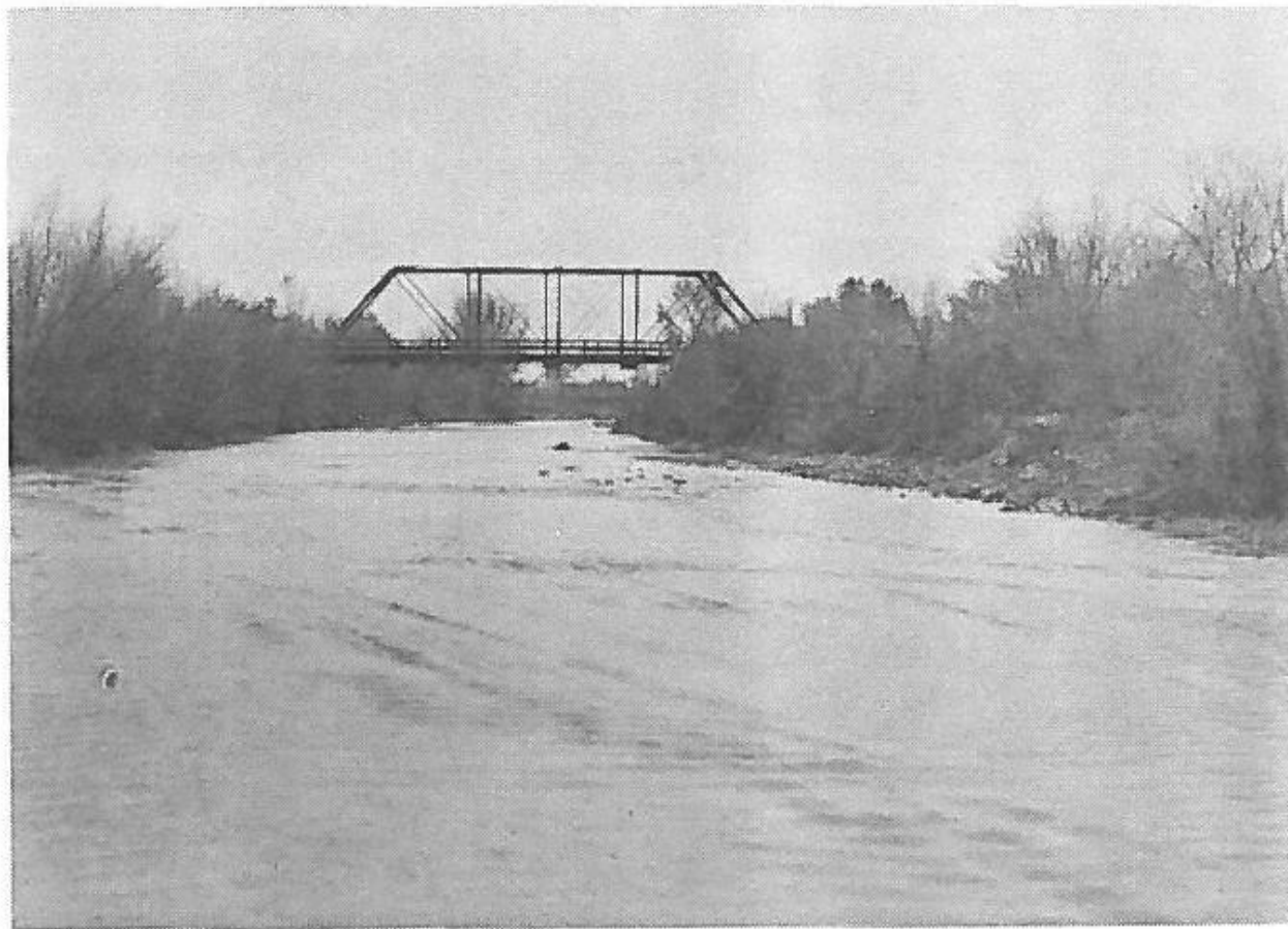
Figure 29. View looking upstream at Congress Street in 1902. The deep arroyo that eroded in 1890 and 1891 made river crossings more difficult. By 1902, a Pratt Truss steel bridge had been erected to span the river at Congress Street. This photograph shows a young stand of willows and cottonwoods that were probably established after the 1890 flood (Arizona Historical Society, Tucson, Negative No. 26698).
