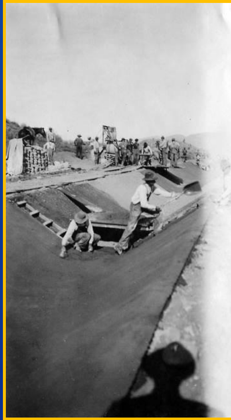
Concrete canal lining project, 1913
