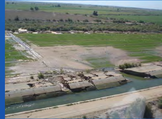
Damage to canal in Mexico from earthquake, April 2010
